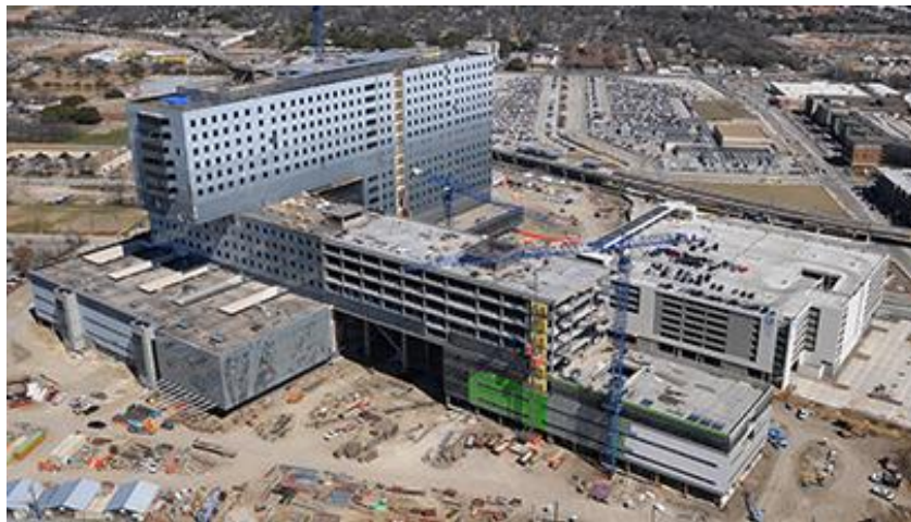
Parkland Hospital under construction
